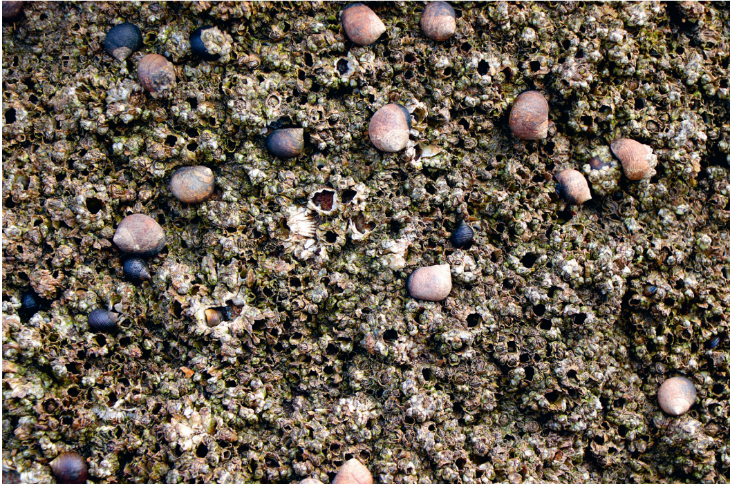
The concrete pylons on Cramond causeway are consumed by nature, and appropriate creatures reveal.
